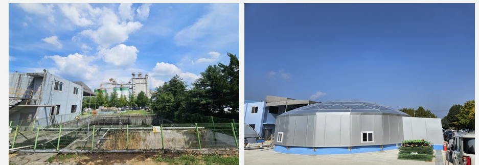
Before construction → After construction
